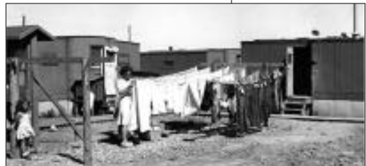
From the top: Housing ranged from eight-plexes to Quonset™ huts to expandable trailers; the interior of a Sundt apartment shows how the owner's belongings could bring a little charm to the apartment; the military personnel fared much worse, however, as this barracks photo shows.
