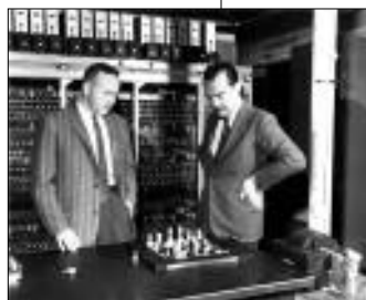
Top: She's a MANIAC — the computer that is. MANIAC was built to solve large-scale hydrodynamic problems.
